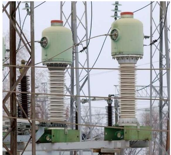
Figure 1: Traditional current transformer
